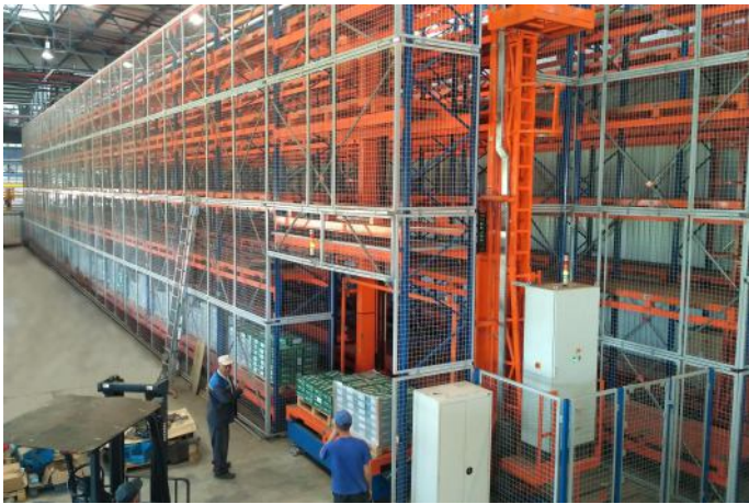
Automated rack-type storage system
